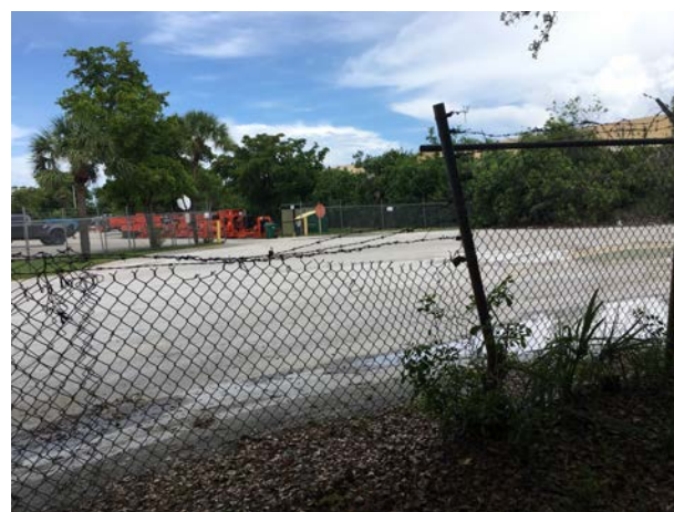
The North boundary is presently the primary access and egress points to the plant on NW 18 th Street. There are two gates openings. Both gates are left open and have been damaged and non-operational. The barbed wire on the top of the chain link fencing has been damaged and not consistent.
